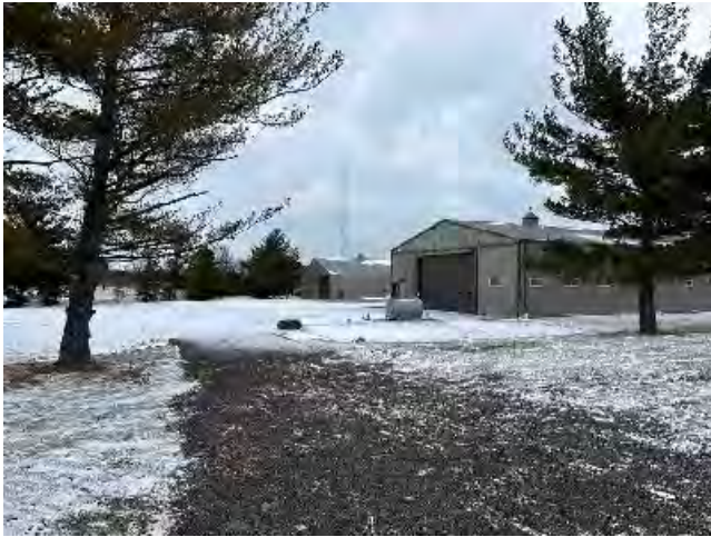
Photo 1: Facing north towards adjoining property. AST on adjoining property in view.
